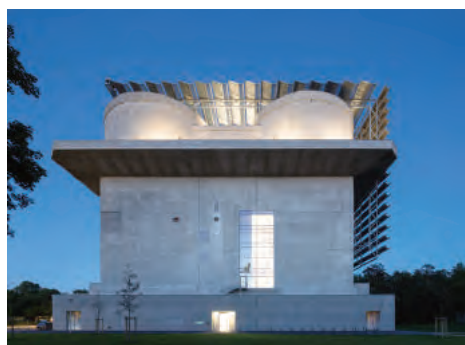
Energy Box of the International Building Exhibition (IBA)
