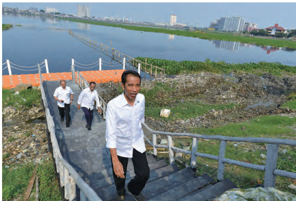
□ Jakarta Residents in the Newly-built Pluit Reservoir
