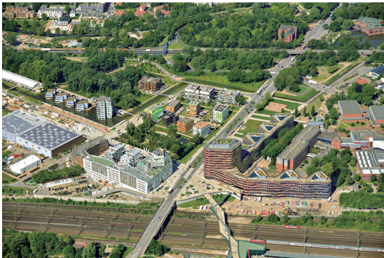
□ Energy and Network Center in Wilhelmsburg, Hamburg
