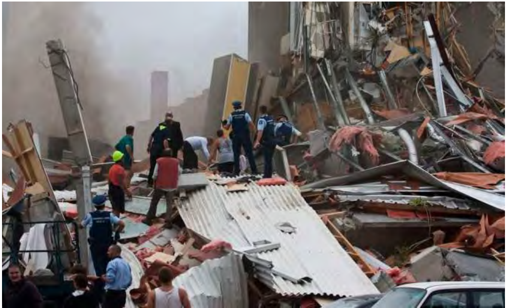
Post-earthquake Site of Christchurch
